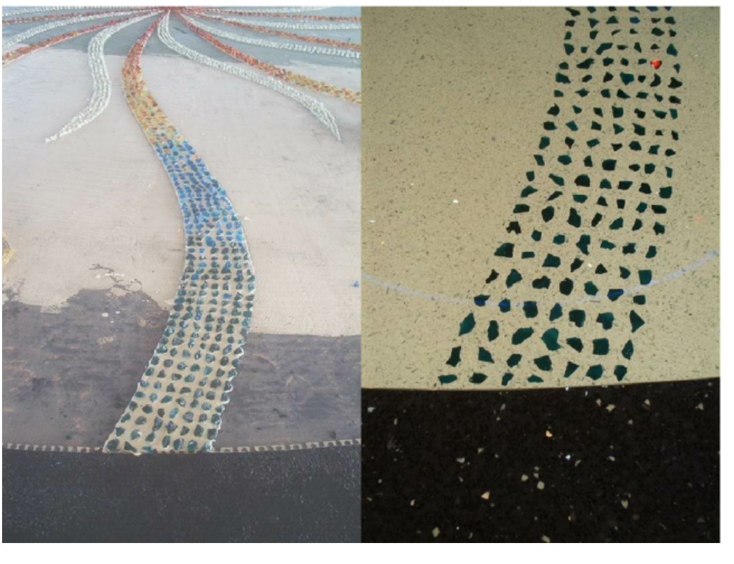
09 EXAMPLES OF AGGREGATE DESIGN FEATURES-DESIGN FEATURES ACHIEVED BY LAYING LARGER AGGREGATE INTO SPECIFIC SHAPES AND IMAGES. AI.114
